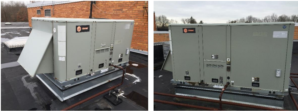
Figure 13-Roof Top Units
